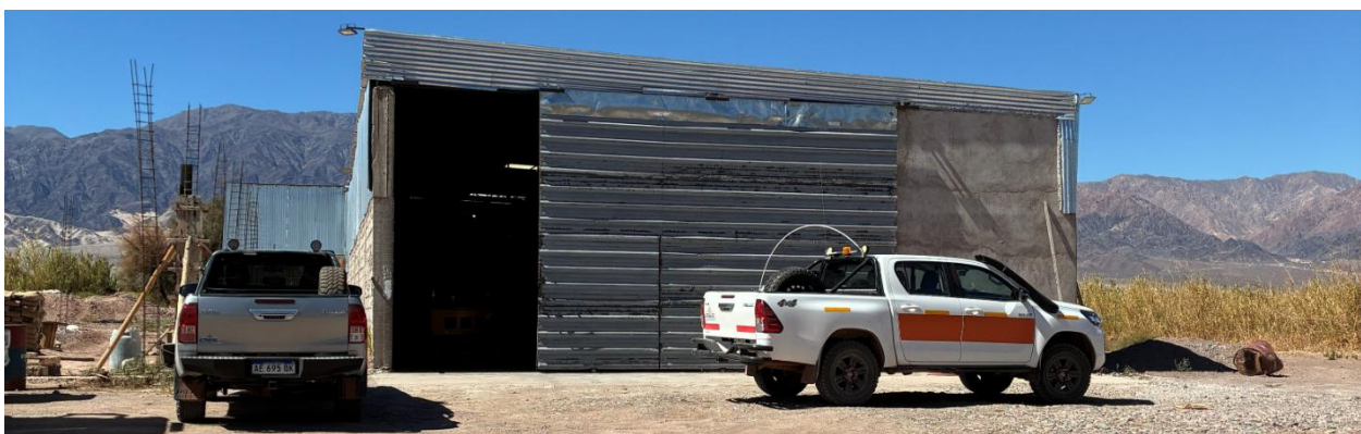
Figure 12-3: Core Storage Facility
